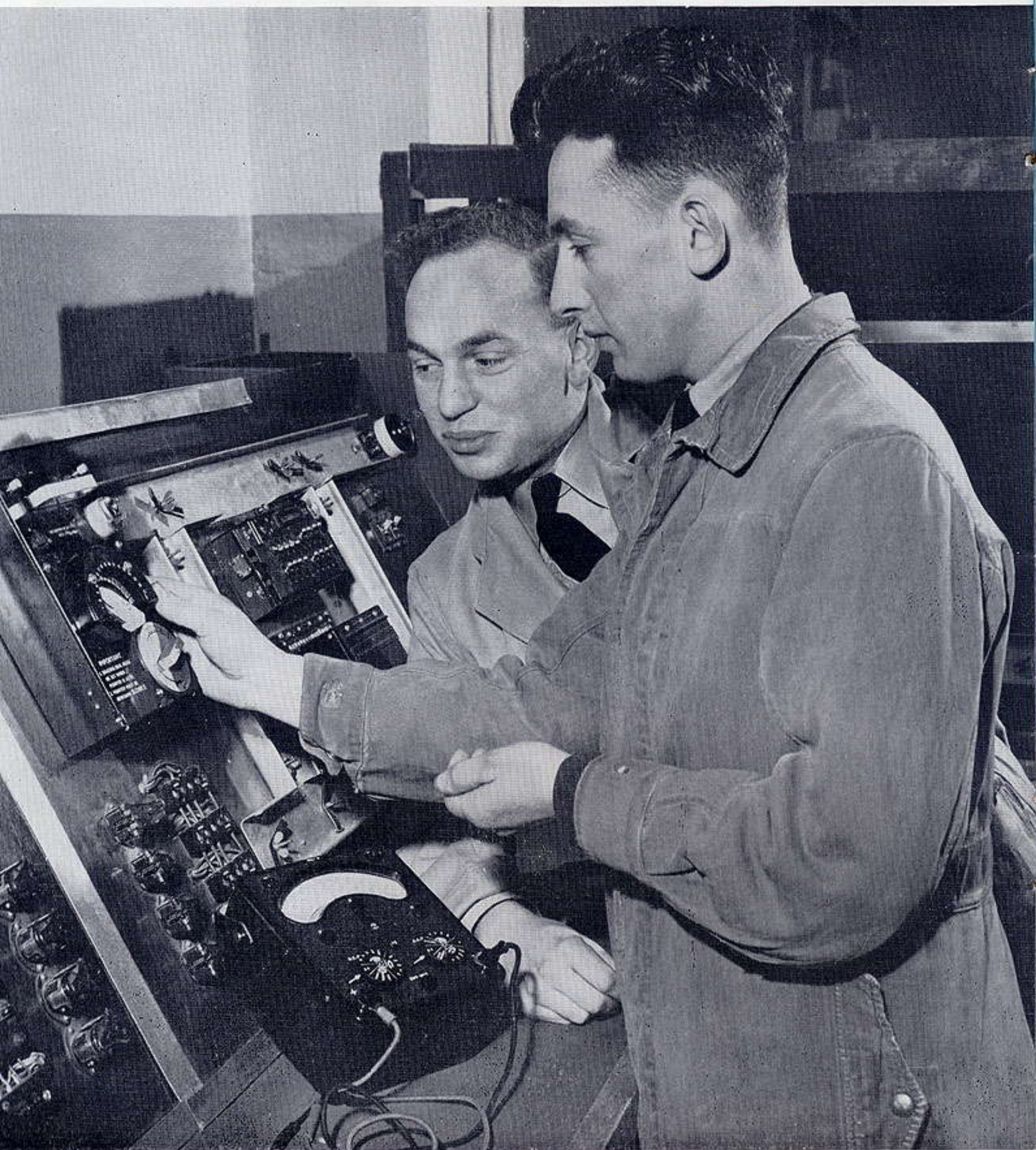
A time check on a bomb-release circuit
