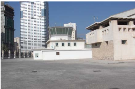
View of the ATC Tower & Guard Tower
